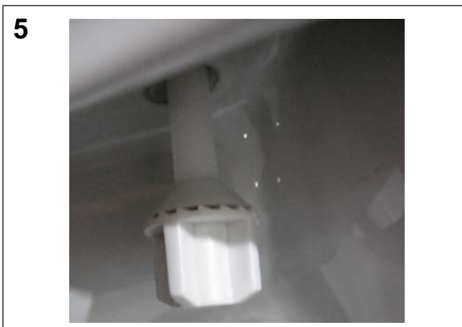
Underneath the pan attach the washers and nuts.
